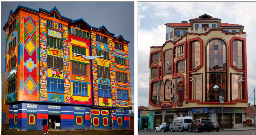
Photograph 7.5. New architectural trends in El Alto
